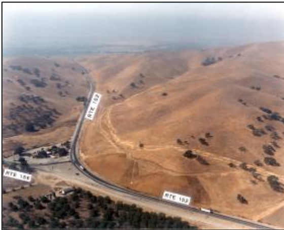
Figure 7: SR 152/156 existing conditions - surface, 2-lane state highways with shoulders
